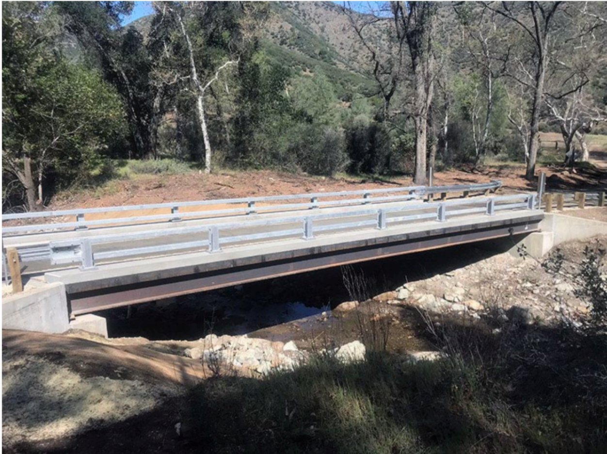
Figure 10. One of two recently constructed bridges over Davy Brown Creek, which replace at-grade road crossings that have impeded steelhead passage. Davy Brown Creek is part of the Santa Maria River watershed, and is tributary to Manzanita Creek and the Sisquoc River, a federally designated Wild and Scenic River. March 30, 2022. Photo: Mark H. Capelli, National Marine Fisheries Service.
