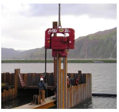
Figure 3. Installing sheet piles with a vibratory hammer.
