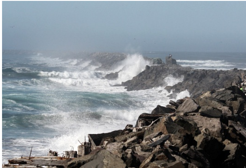
Figure 20. Photograph of the South Jetty in September.
