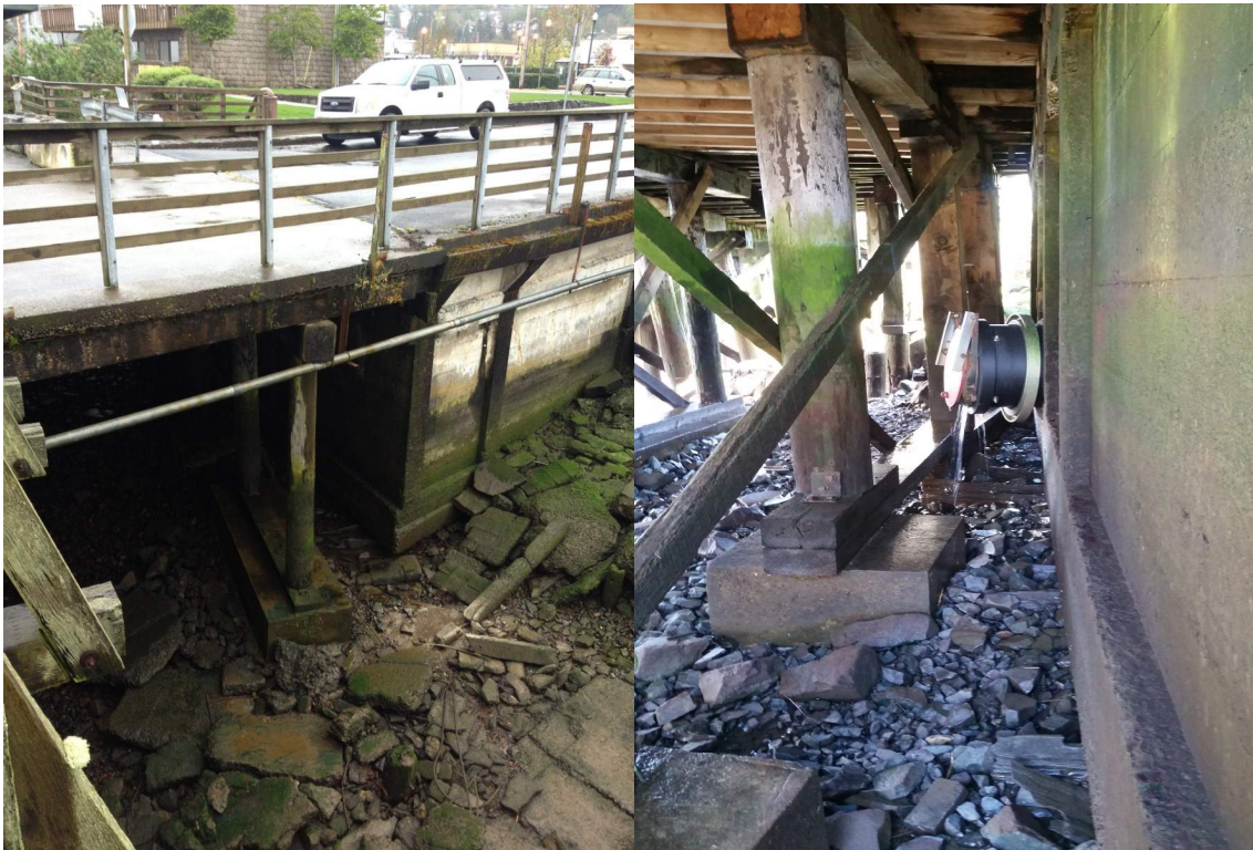
Photographs of existing concrete footings that will need to be removed during demolition activities
