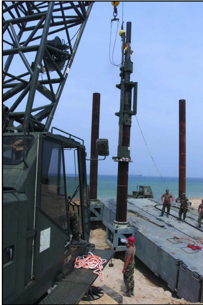
Figure 1-4. Pile Driving During ELCAS (M) Construction
