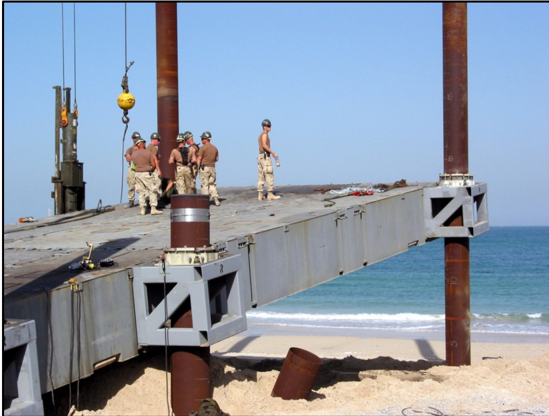
Figure 1-3. Assembly of Pier Connection on Beach
