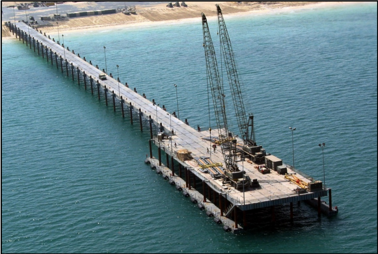
Figure 1-5. Navy Elevated Causeway System, Modular
