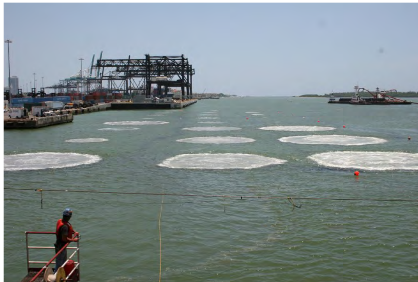
Figure 5 - Typical rectangular blast pattern (Miami Harbor)
