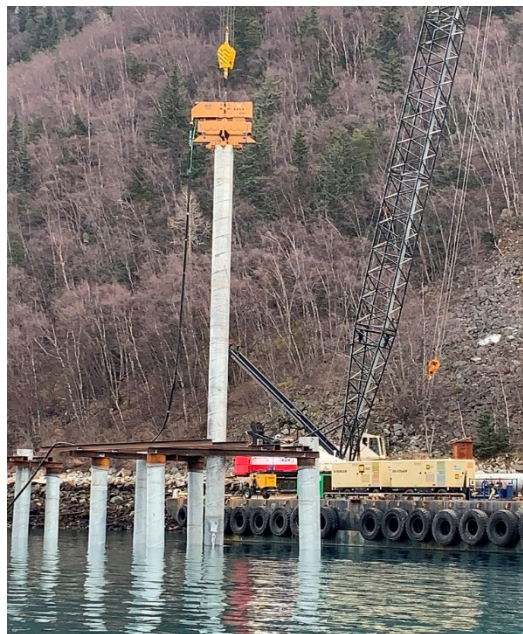
Figure 3. Vibratory hammer on pile.
