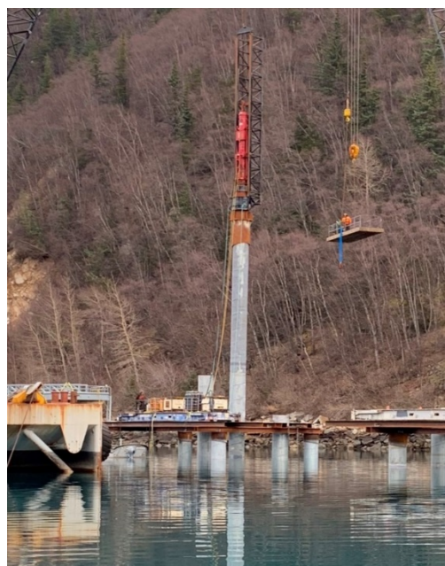
Figure 4. Impact hammer on pile MD4-V (note drilling shoe).
