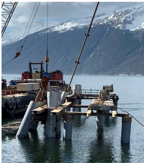
Figure 6. Rock anchor casing installation for pile MD4-NE.
