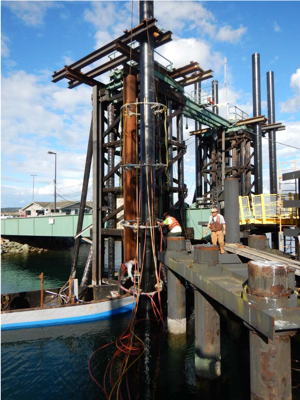
Figure 1 Preparing Bubble Curtain
