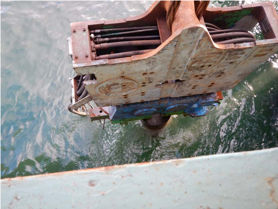
Figure 7 Vibratory Removal of Steel Pile
