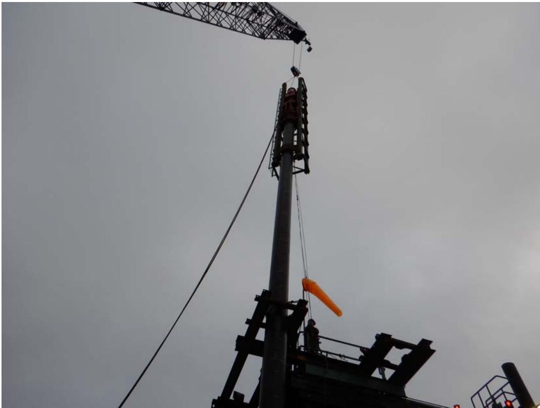
Figure 2 Positioning Impact Hammer
