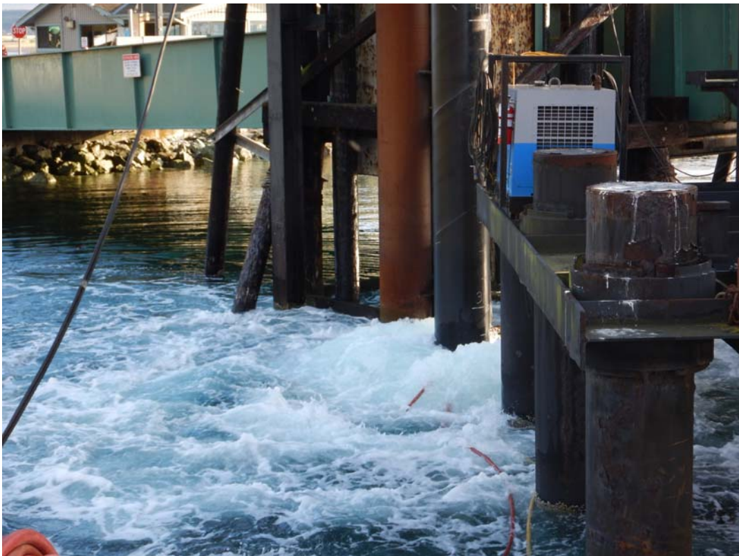
Figure 3 Bubble Curtain Active
