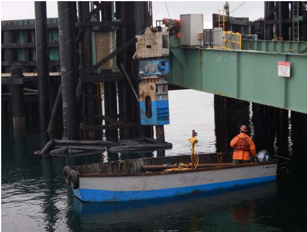
Figure 5 Vibratory Removal of Timber Pile
