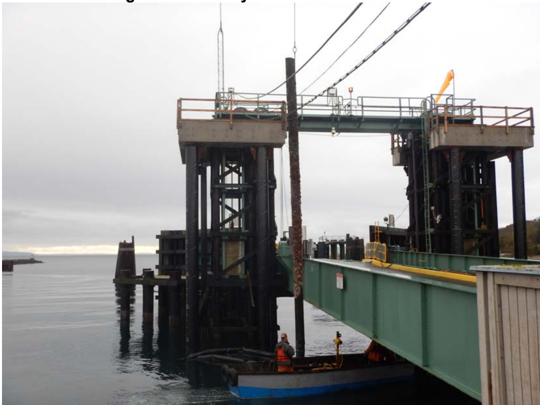
Figure 6 Cable Lift Timber Pile to Barge
