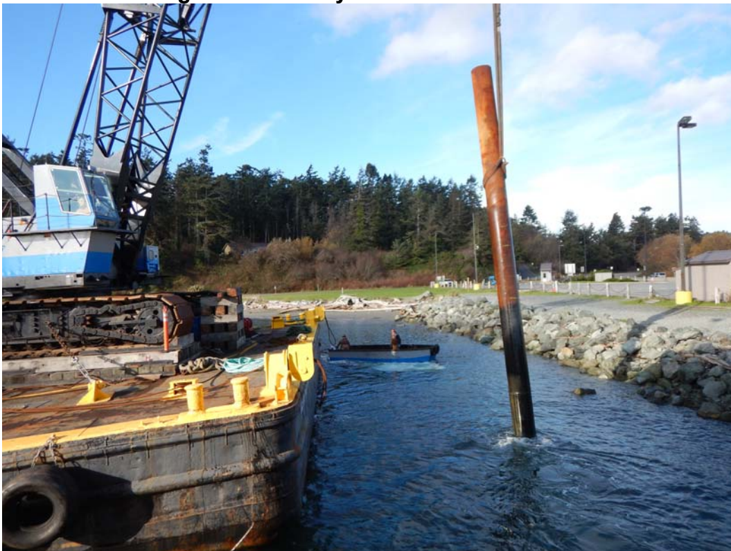
Figure 8 Cable Lift of Steel Pile to Barge
